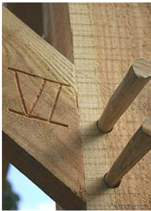
Figure 1: Timber framed building joint.
