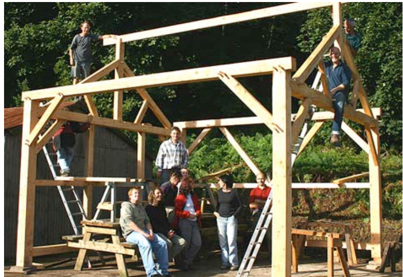
Figure 2: Timber framing course, Derbyshire 2006.
